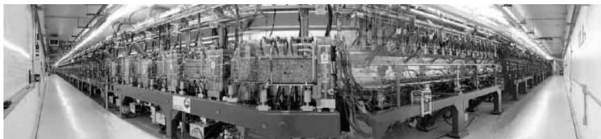
Figure 8.4 Magnets in the storage ring at the SNS (courtesy of the Oak Ridge National Laboratory).
